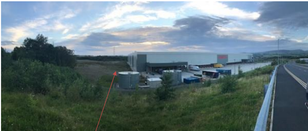
Photo 1 – the application site on the southern elevation of the existing building
